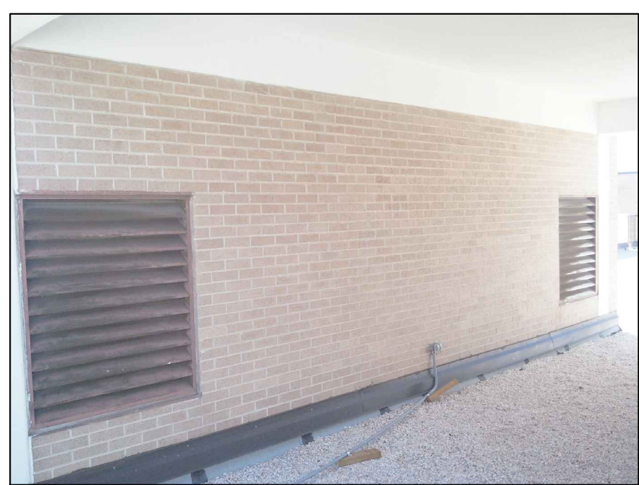
③ EXISTING HOISTWAY VENTS
